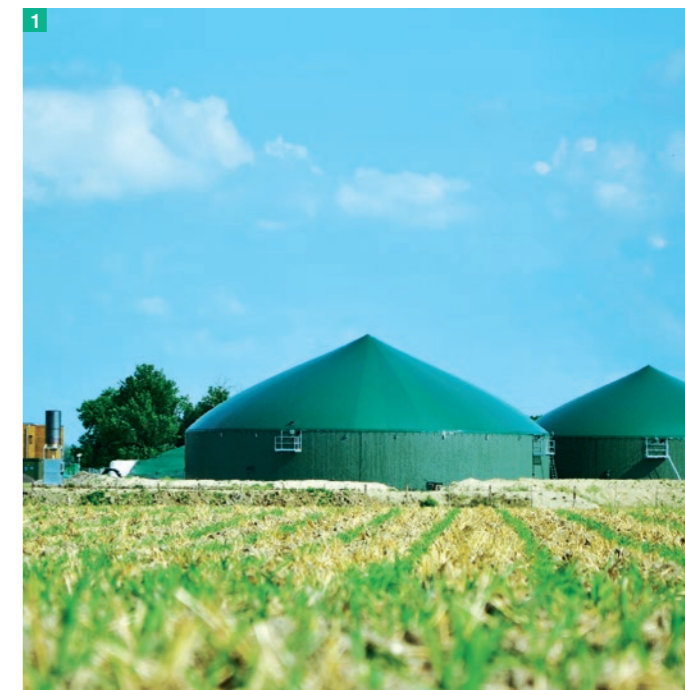
The Bassée Biogaz anaerobic digestion unit in Noyen-sur-Seine
