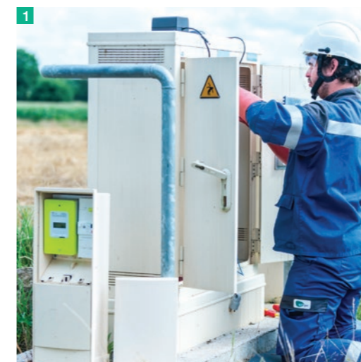
1 Work on electrical box
